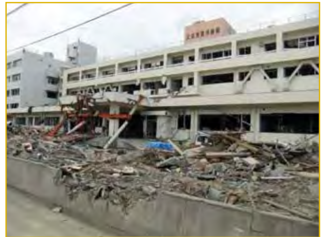
Fig. 2 Everything on the 1st floor to the 4th floor was destroyed by the tsunami. Only those on the 5th floor survived.
